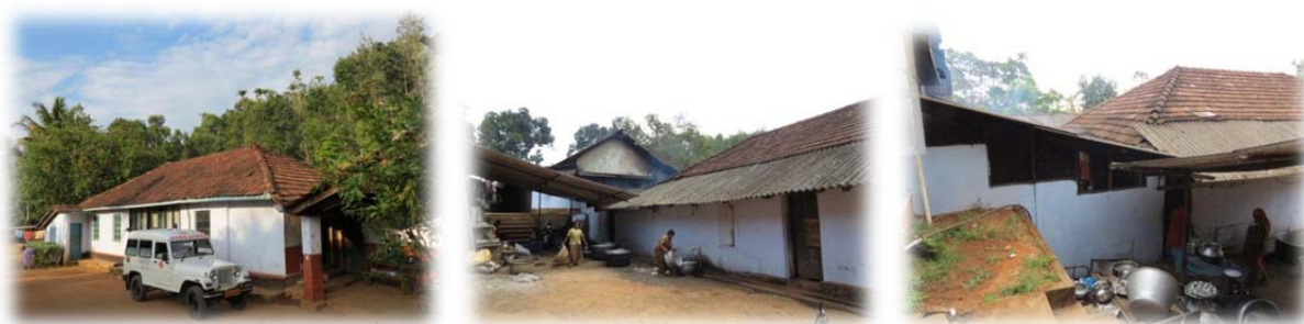
Photos: Old clay farmhouse (main entrance, back elevation and current kitchen).
